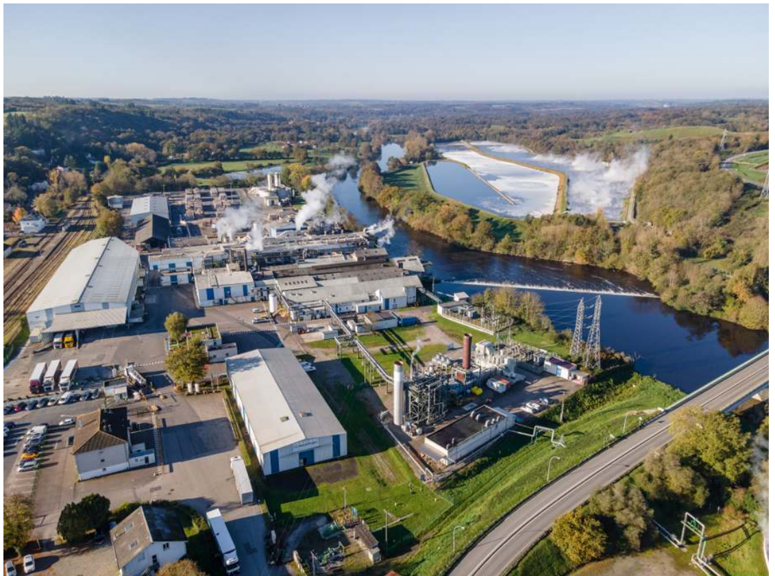
The integrated industrial power-to-hydrogen-to-power solution with a gas turbine type SGT-400 at Smurfit-Kappa, Saillat-sur-Vienne, France (Courtesy: Engie)
