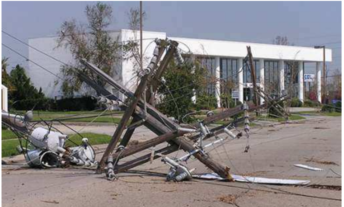
Aftermath of the storm
