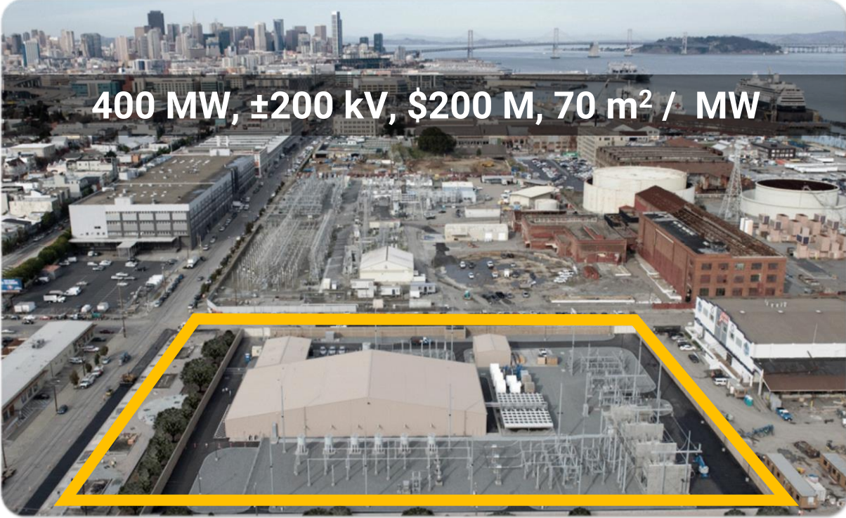
Trans Bay On-shore HVDC Station (2010)
