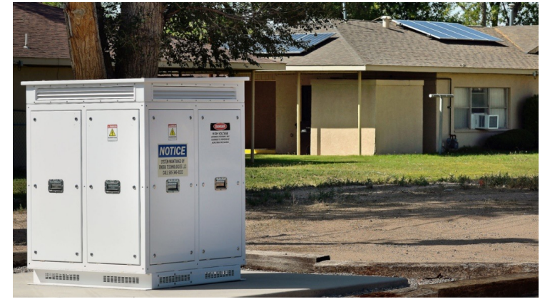
BlockEnergy Nanogrid Serving Residential Housing Loads
