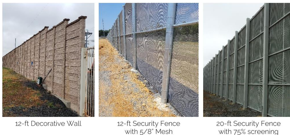
Figure 3: Substation Perimeter Fence Options.
