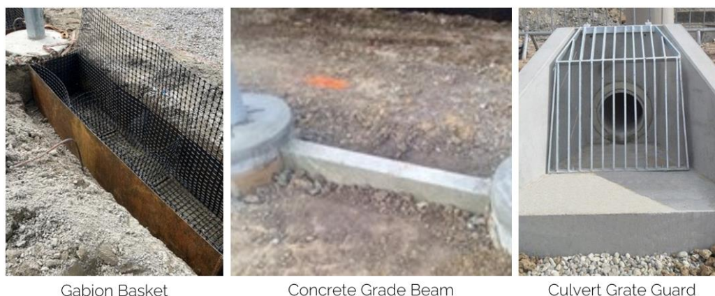
Figure 4: Substation Perimeter Fence Anti-Dig Options.
