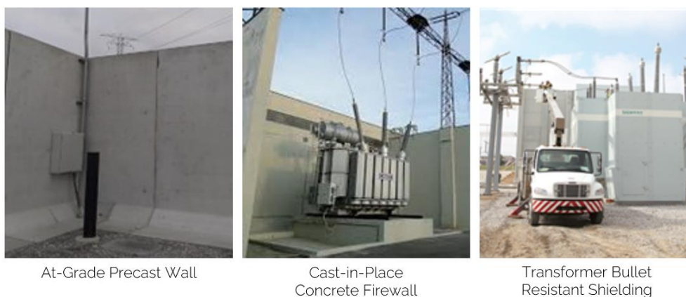
Figure 6: Substation Transformer Protection Alternatives.
