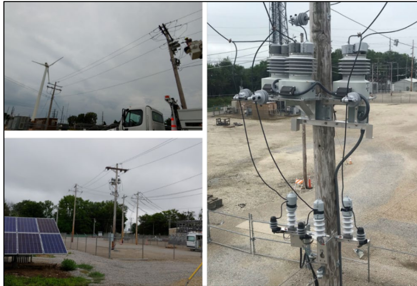
Figure 3: Renewable energy sources at the microgrid and field installation of voltage sensors
