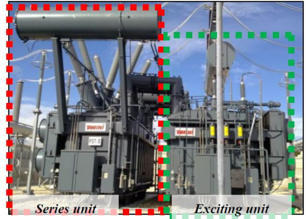
A2-207_2014: New Phase Shifting Transformers in the Italian Transmission Network - Design, Manufacturing, Testing and Electromagnetic Transients Modelling
