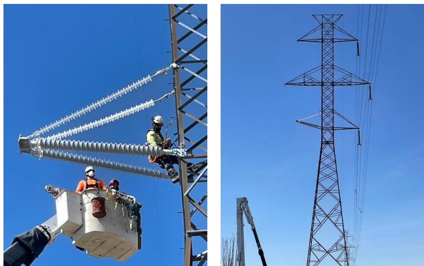
Figure 16. Trail fit of retrofit composite insulated cross-arm.
