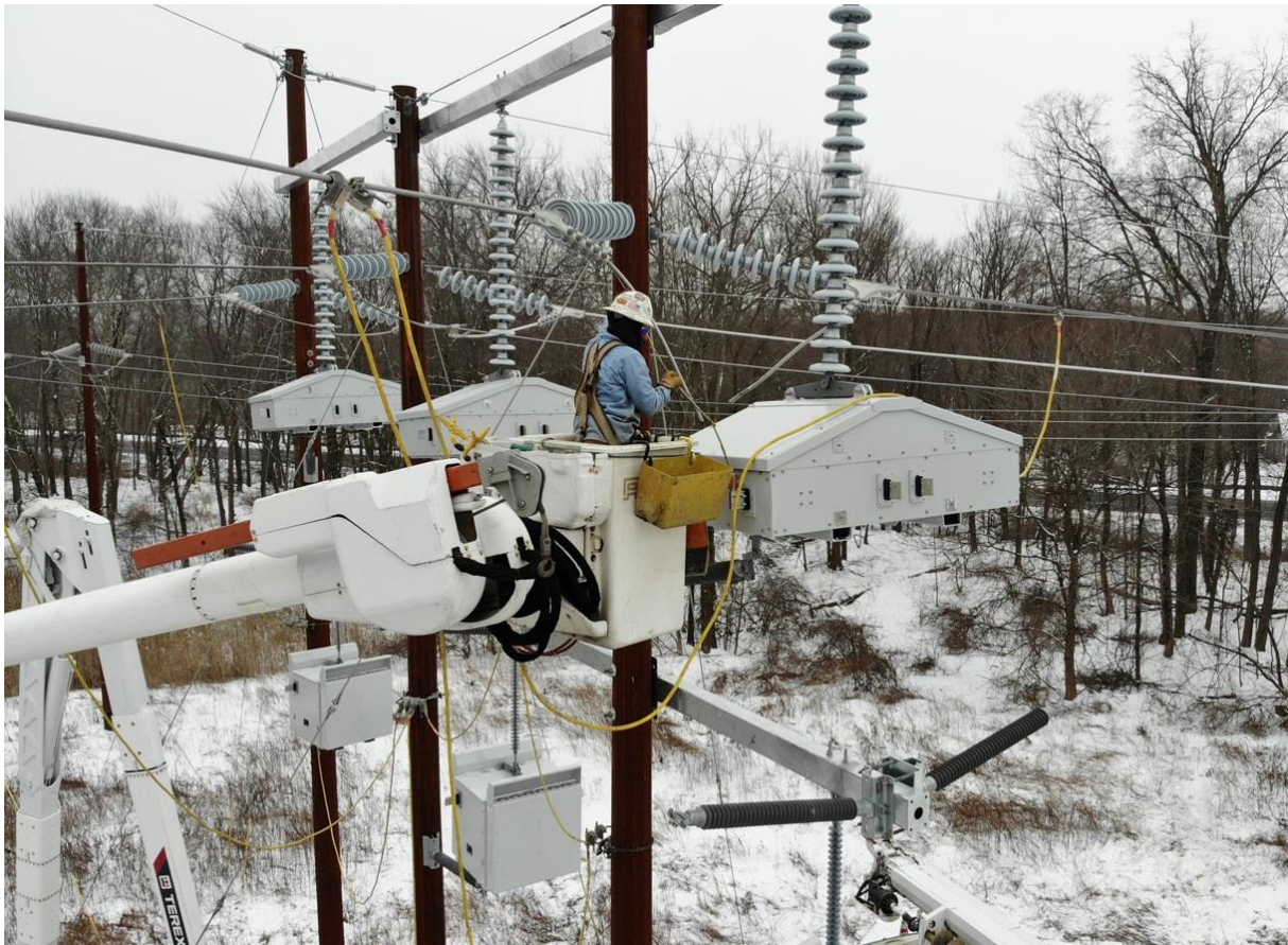
Figure 4: Installation of M-SSSC Phase 1 Pilot on Central Hudson's system
