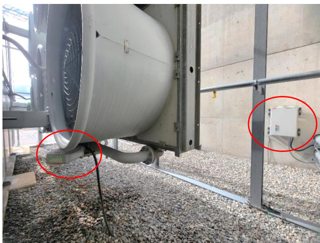
Figure 1: Image showing the location of the CoreSense Sensor Head (left) and the CoreSense Analytical Unit (right) installed on one of the six converter transformers.
