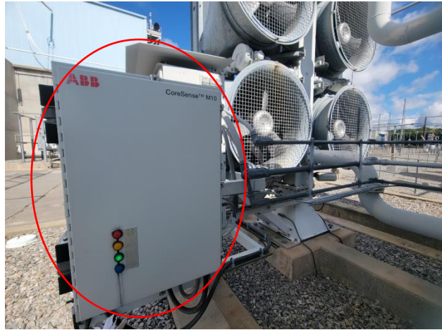
Figure 3: Image showing the location of the the CoreSense Analytical Unit (left) and the CoreSense Sensor Head (right) installed on one of the three station reactors.
