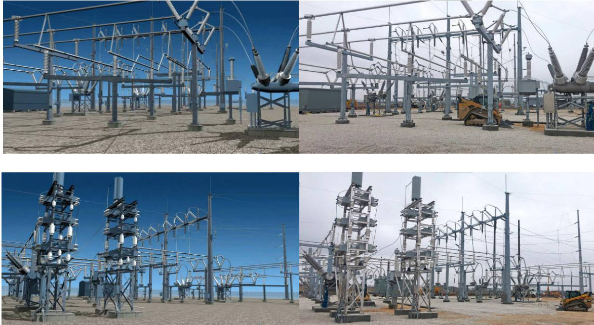
Figure 1. Comparison of Design Digital Twin Model and Actual Construction (Model : Left, Constructed Station : Right)
