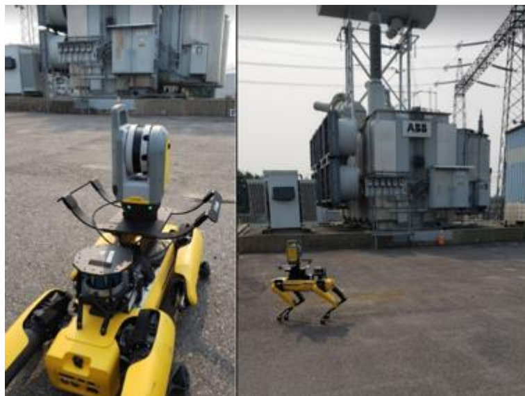
Figure 1: Images of the robot with the attached Trimble X7 payload while scanning the area of the converter transformer.
