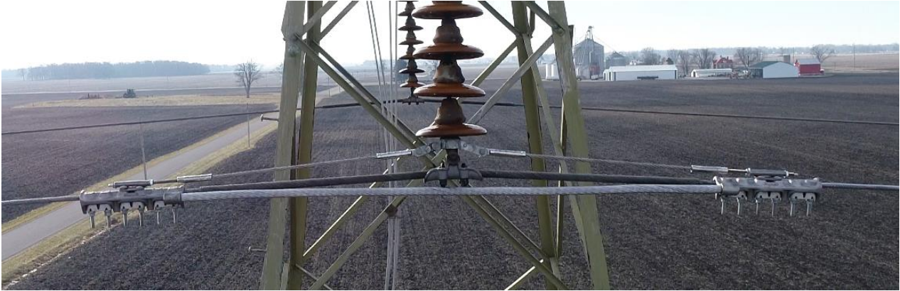
Typical BallCap application, 115 kV 477 Hawk with armor rods – broken strands under rods
