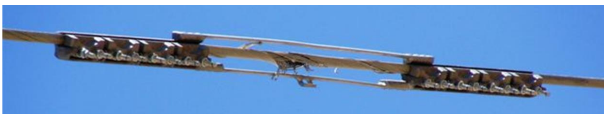
Gunshot damage restored using an EEMS designed for splice mitigation.
