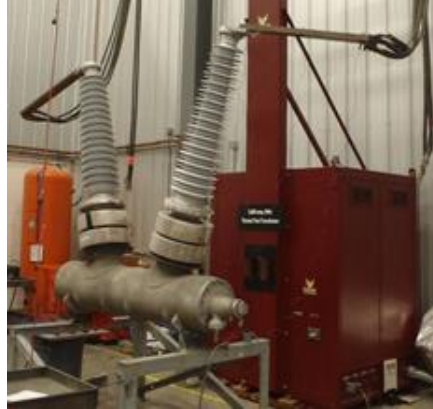
Figure 6: DT1-145g during temperature rise test at 3000 and 4000 A.
