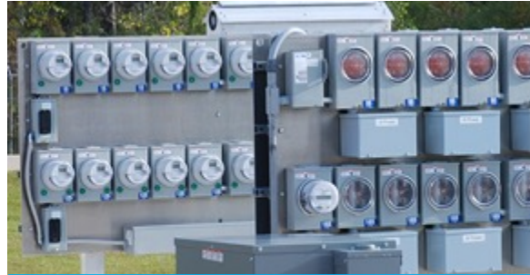
1. AMI (Advanced Metering Infrastructure)
