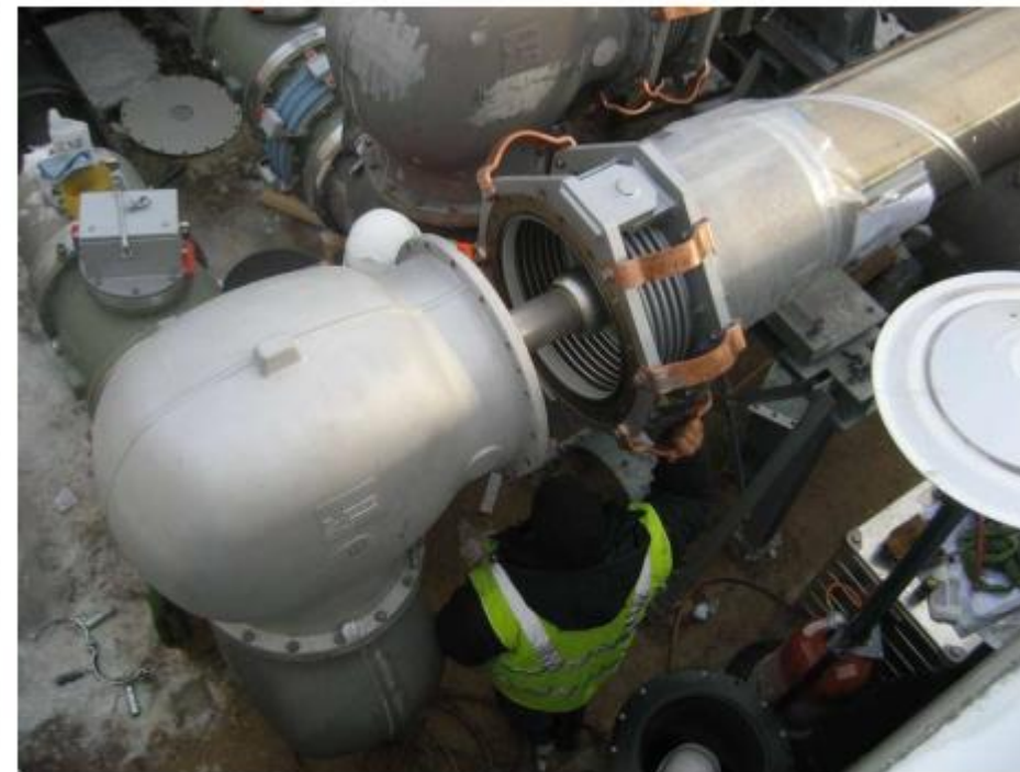
Coupling of male and female sliding contact
