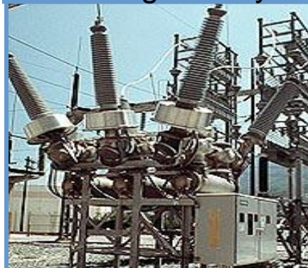
Dead Tank Switchgear Bay
