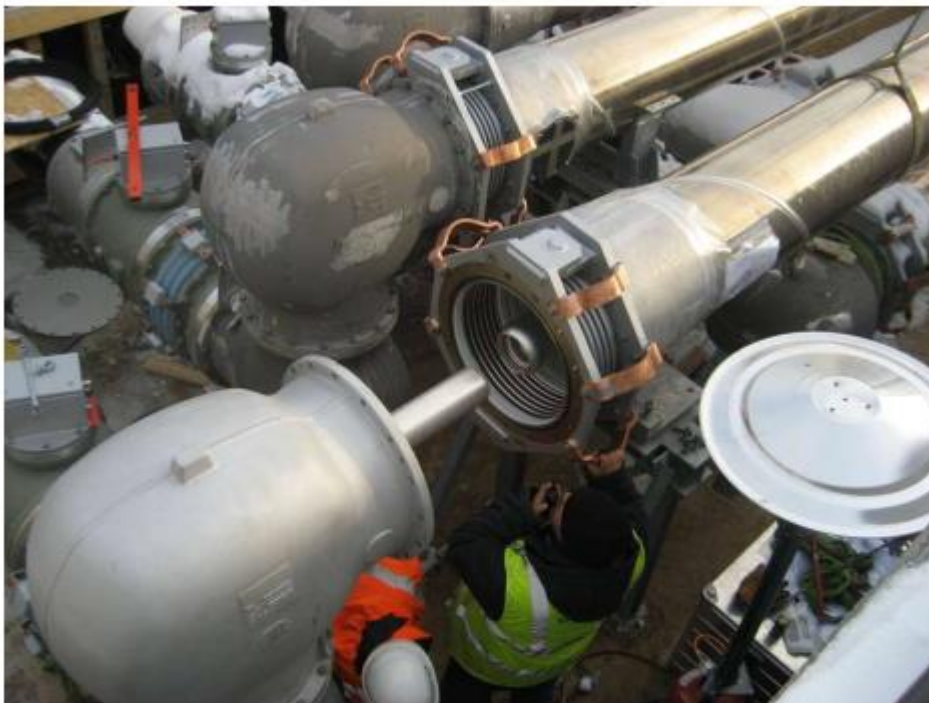
Connection of elbow module and expansion joint
