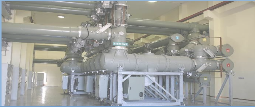
Gas-Insulated Switchgear GIS
