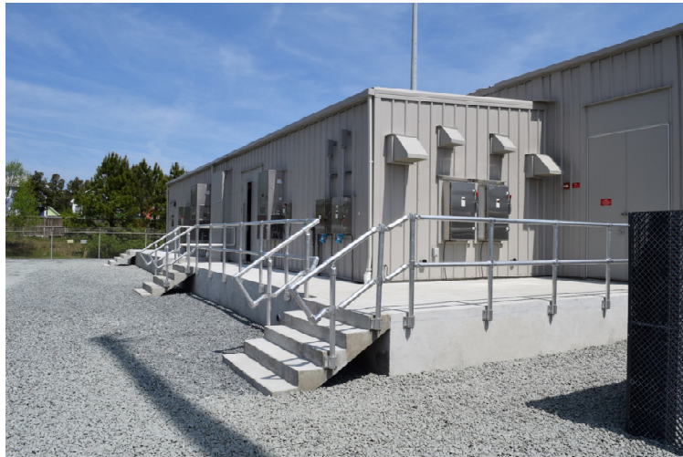
Fig. 4. Colington STATCOM control building with raised platform
