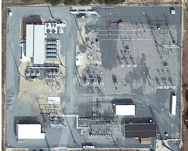
Fig. 5. Colington substation with new STATCOM
