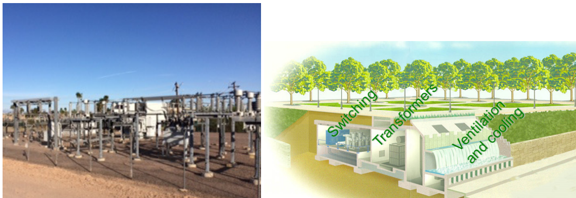
Figure 5 – Traditional AIS versus Resiliency Enhanced GIS
