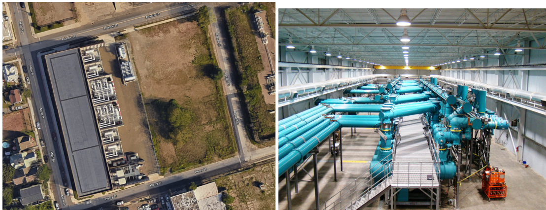
Figure 5 – Traditional AIS versus Resiliency Enhanced GIS
