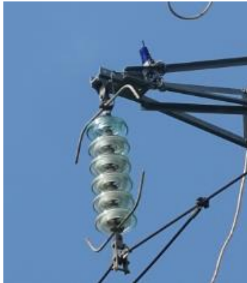
Figure 11: Overall smart insulator device arrangement.
