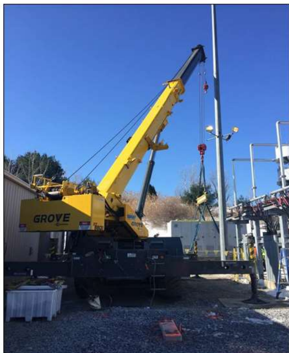
Lifting Inverters into the building (26,000 lbs each)
