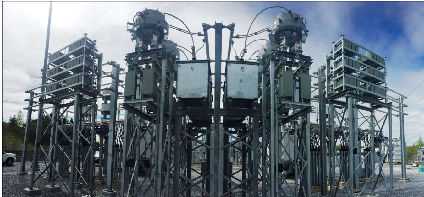
STATCOM Harmonic Filters Arrangement
