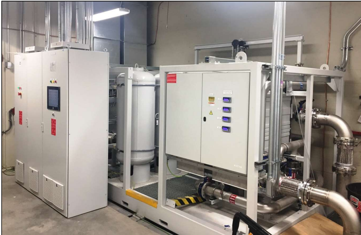
STATCOM #1 – Cooling Skid & Hoist Mechanism for Maintenance
