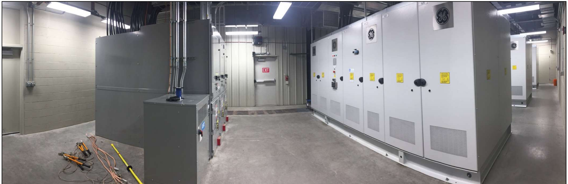
STATCOM #1 – Inverters and 3.2kv Switchgear
