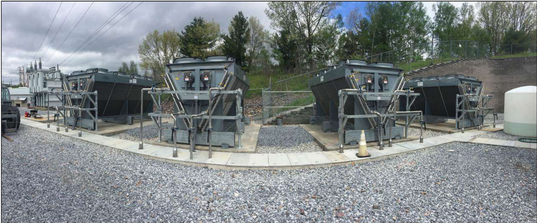
Cooling System – Outdoor Heat Exchangers
