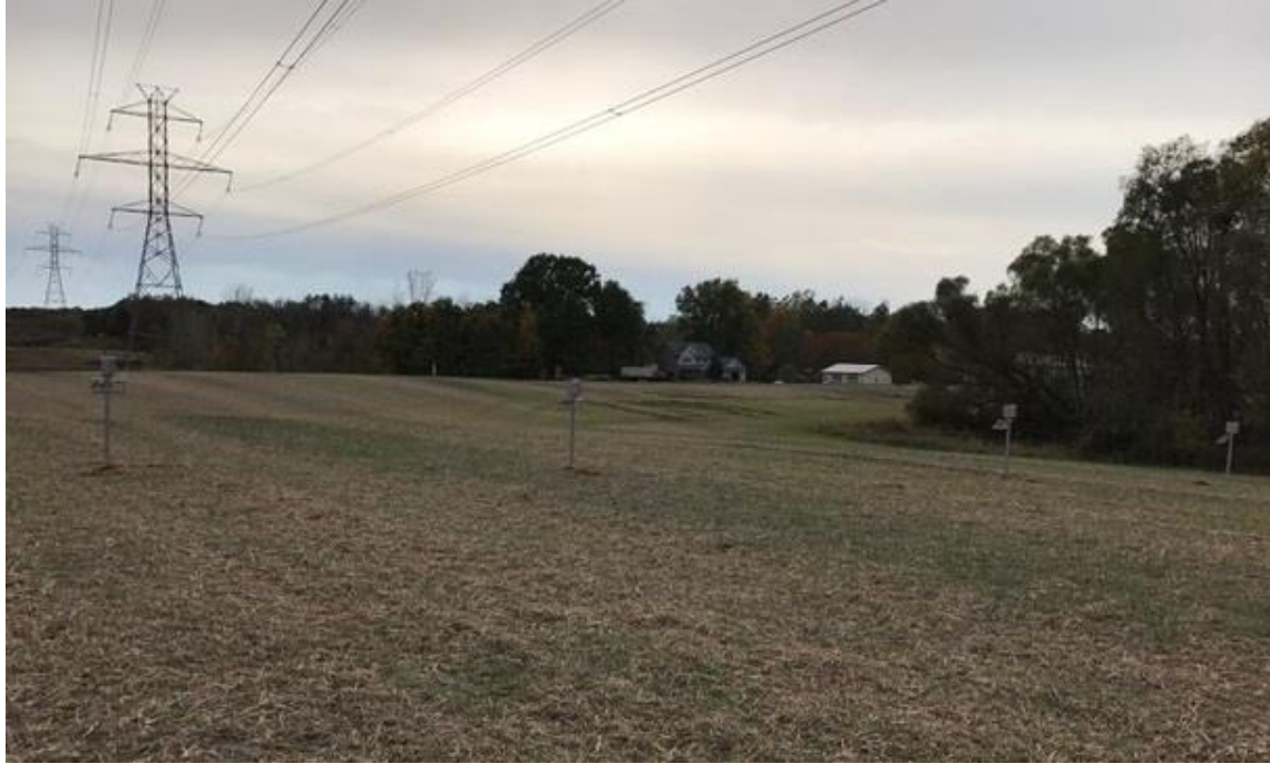
LineVision monitor array at installation Site 3 of 3
