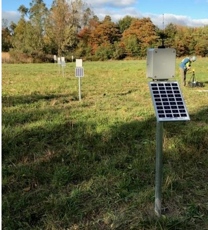
LineVision monitor array at installation Site 1 of 3
