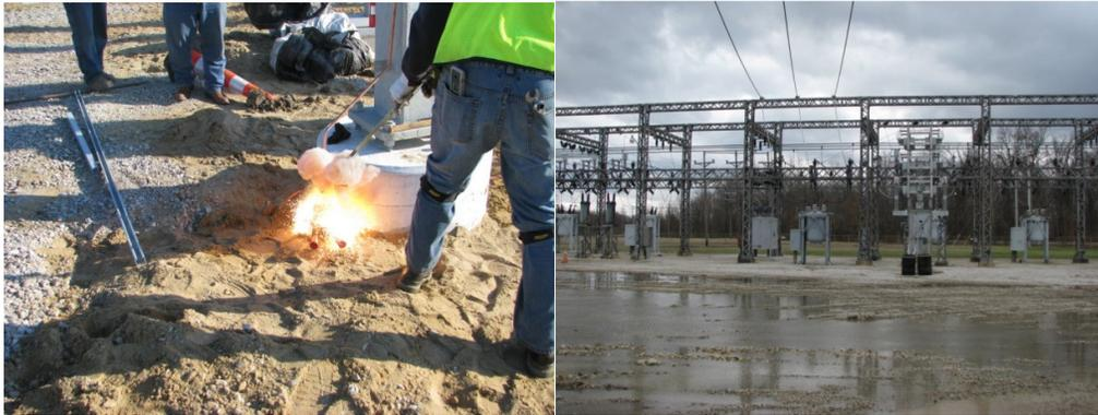
Fig. 6. Exothermic weld ignition (left) Challenging site condition (right)
