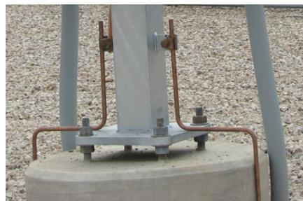
Fig. 3. Two ground connections for one structure
