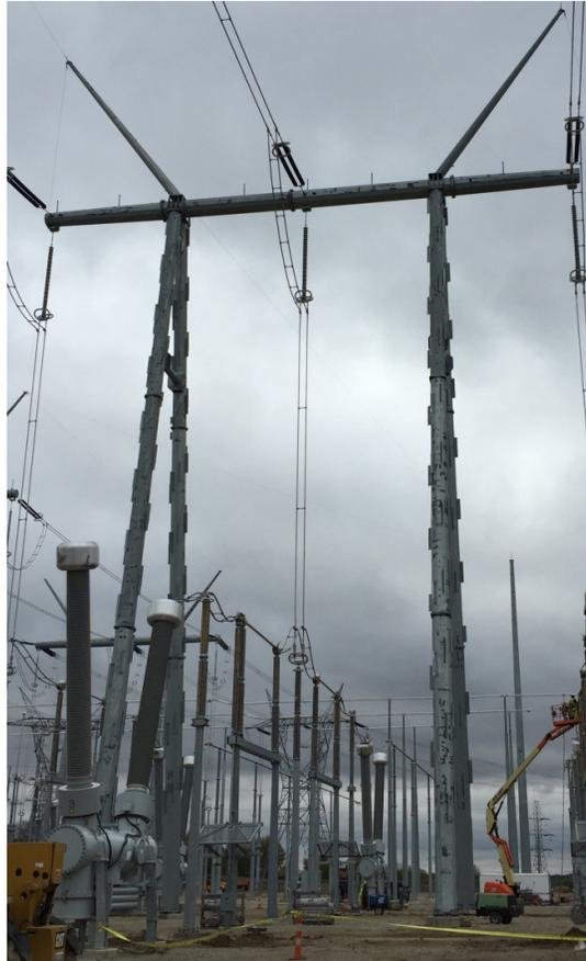
Fig. 5 Retrofitted dead-end structure with strakes
