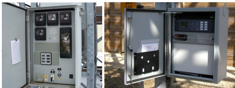
Figure 3 Electromechanical and microprocessor-based relays in the yard
