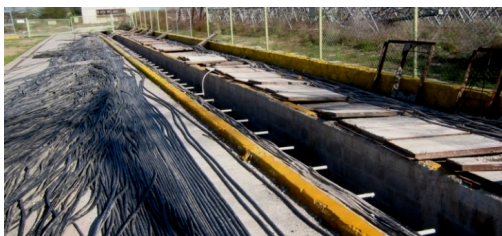
Figure 6 Refurbishment project showing the amount of copper wire replaced with fiber-optic-based I/O module technology
