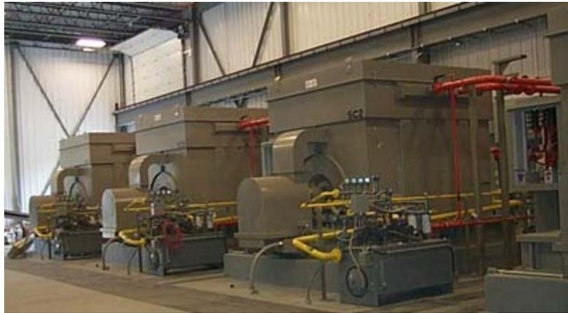
**Figure 2. New synchronous condenser project in New England (Source: GE/VELCO/IEEE)**
