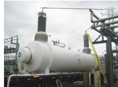
Figure 1: 138kV Class HTS-based FCL
