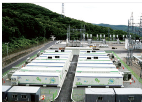
Figure 6: KEPCO deployment of BESS at the Shin-Yongin substation where 16 MW system designed and implemented by EN Technologies is installed.
