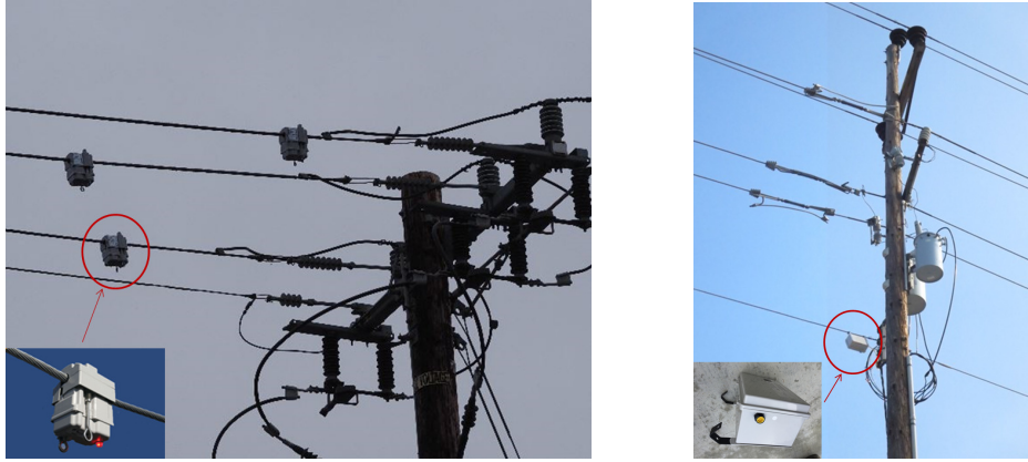
Figure 1: Sensors and monitors to capture fault data. (Left) line sensor, (right) voltage sag monitor
