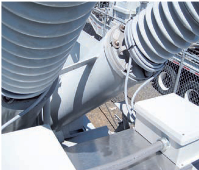
Fig 2: Example optical CT showing freedom to mount in different orientations (Shown horizontally-mounted here)
