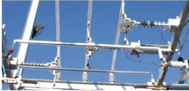
Fig 2: Example optical CT showing freedom to mount in different orientations (Shown horizontally-mounted here)
