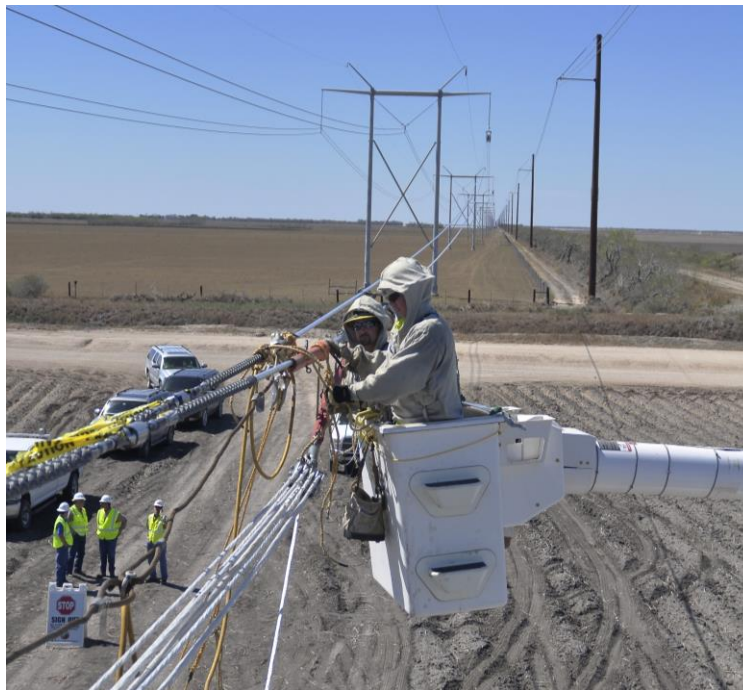
Figure 11 – AEP / Quanta live line 345 kV reconductoring project using ACCC conductor
