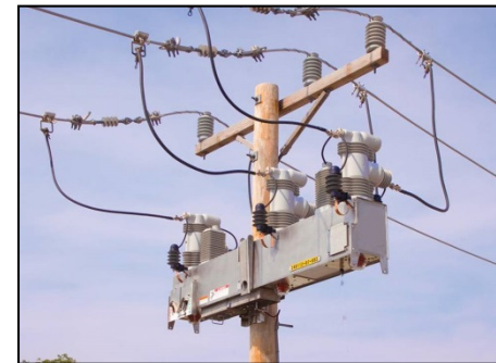
IntelliRupter: Self Powered, Self Contained, Fault- Interrupting Switch
