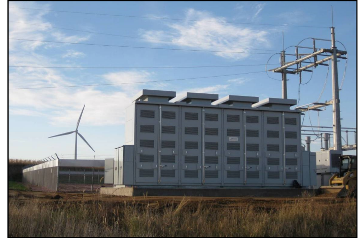
Luverne, MN NaS Battery Installation 1.0 MW for 6 hours Used for wind farm smoothing to facilitate dispatched wind and peak shaving
