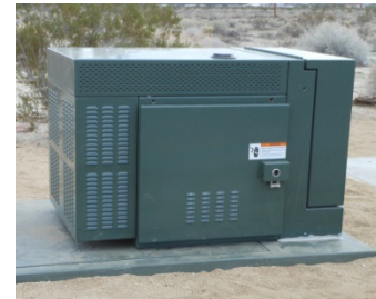
Community Energy Storage 25 kW; 50 kWh Lithium-Ion
