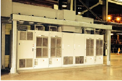
Fig. 3. EX2100e Excitation System for Unit 5 Located on the Turbine Deck
