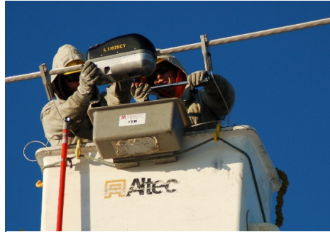
Figure 5: Live line installation of sensor
