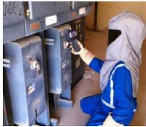
Figure 2: PD measurement on switchgear with anti-arc flashing clothing
