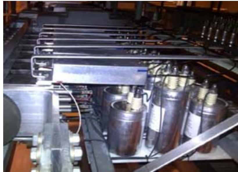
Note: New TCU's and SF6 Filled Snubber Capacitors
