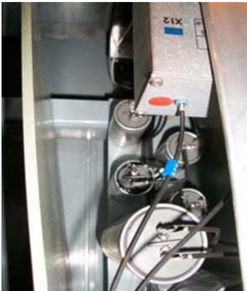
Note: Oil Filled Snubber Capacitors
