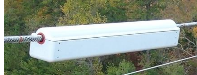
The PowerLine Guardian (formerly known as the Distributed Series Reactor or DSR) injects magnetizing inductance to increase line impedance and “push” power to parallel lines.
