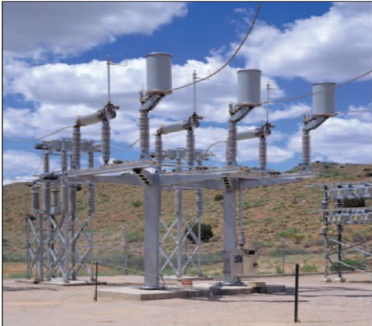
Pre-insertion inductors mounted on 138-kV Vertical-Break Style Mark V Circuit-Switcher.
